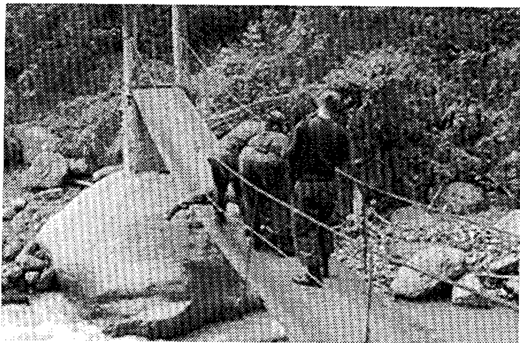
Colombia accused Venezuelan soldiers of blowing up a footbridge on the border
